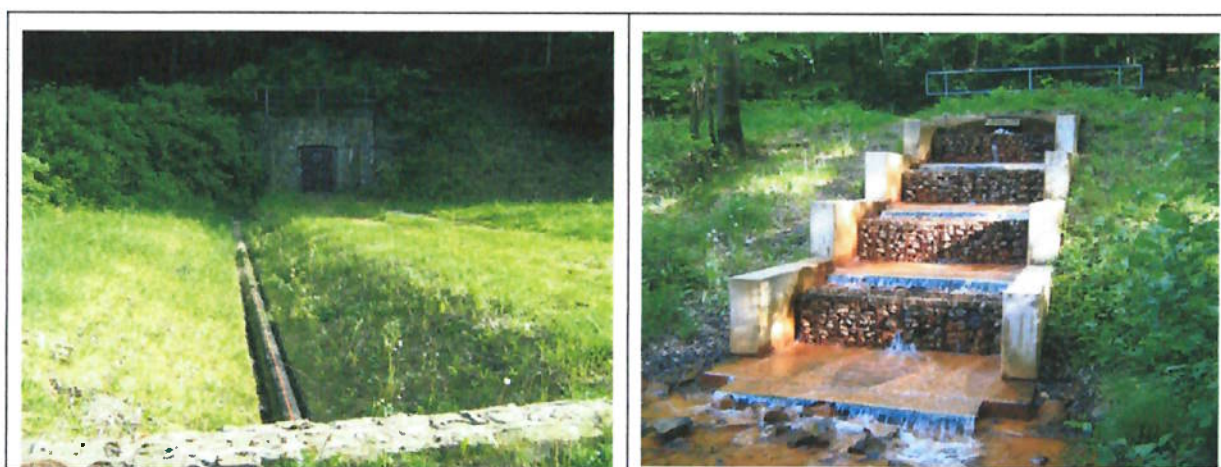
Figure 89: Current situation at the fluorspar mine site: adit with mine water outlet (left); aeration zone for mine water passive treatment of the drainage water (right)
