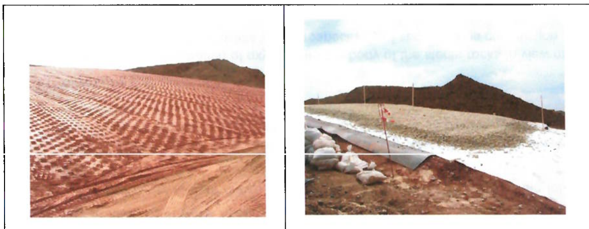
Figure 94: Installation of soil cover systems
