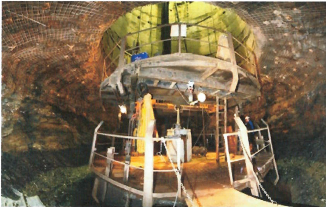
Figure 82: Break out of shaft, preparation for plugging
