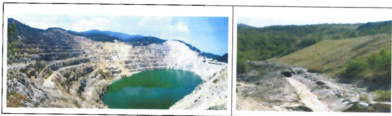
Figure 41: Sample of a flooded copper mine in Bulgaria (left); water diversion channel upstream the mine (right)
