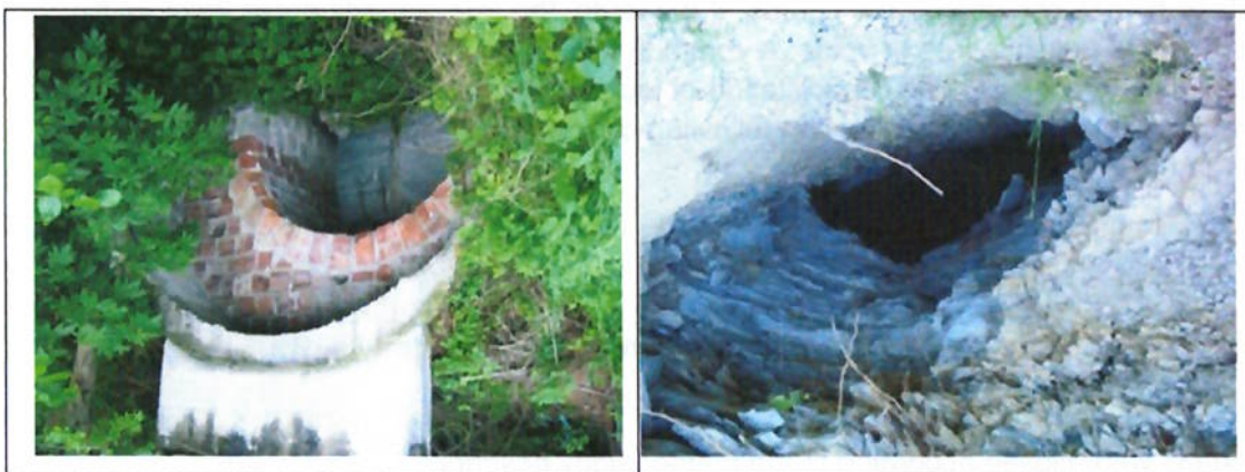
Figure 83: Adit open, no water discharge (left); adit open, water discharge (right)
