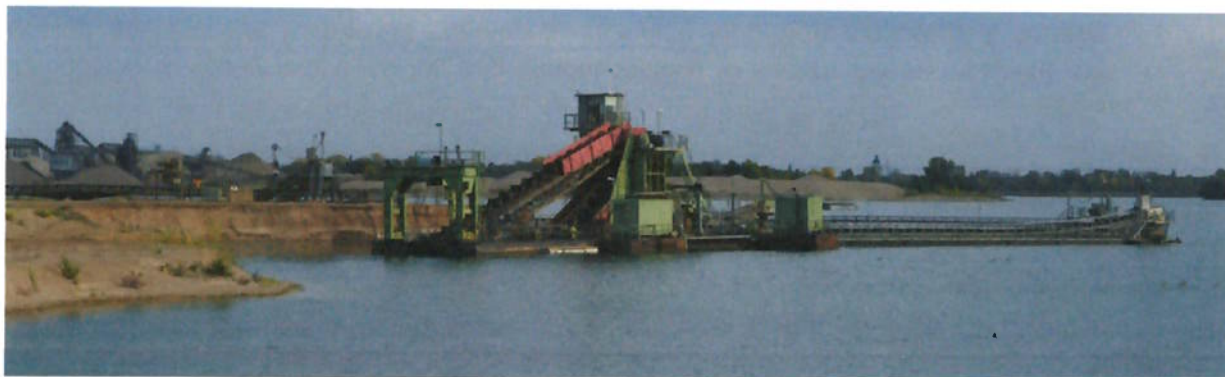
Figure 21: Example of a sand dredging facility
