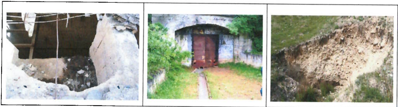
Figure 44: Sample of shafts (left); adits (centre) and sinkholes (right) before rehabilitation
