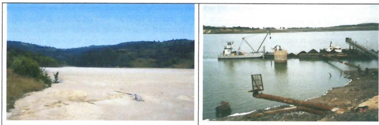
Figure 51: Overview on active tailings pond (left); tailings pond under forced consolidation through subaquatic fill of extractive waste through hopper barge (right)
